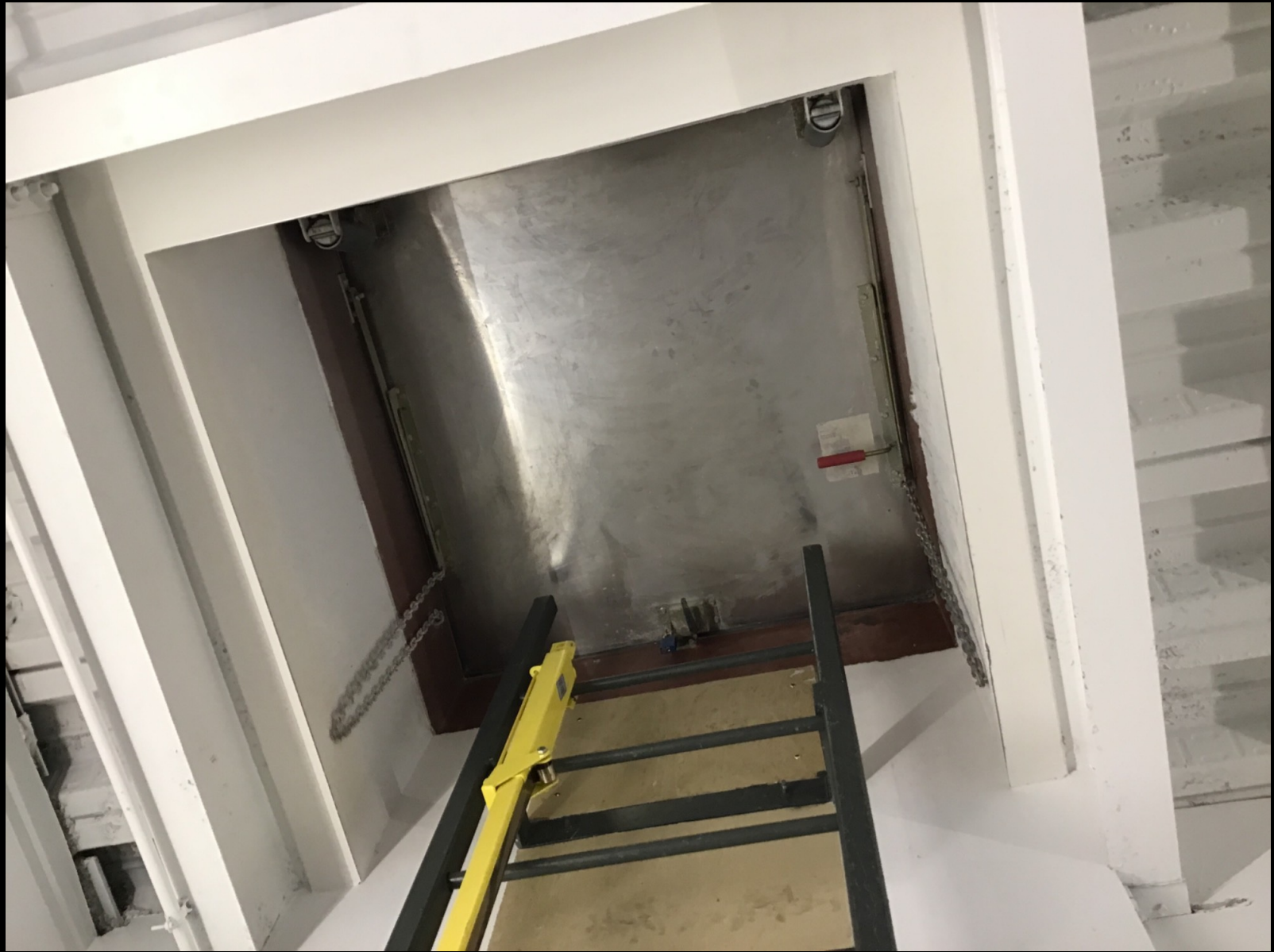
After leaving the roof, we made sure the hatch was closed tightly.
