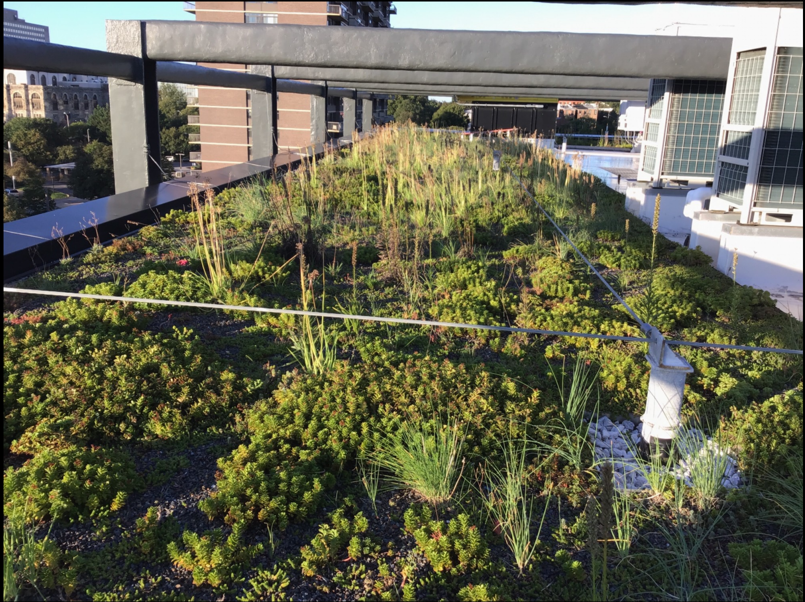
We arrived today to conduct a routine Stewardship visit. The green roof is in healthy condition.
